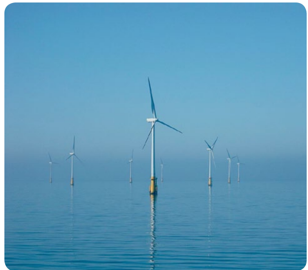
Barrow Offshore Wind Farm – Offshore-Windpark in der Irischen See. Quelle: wikipedia
